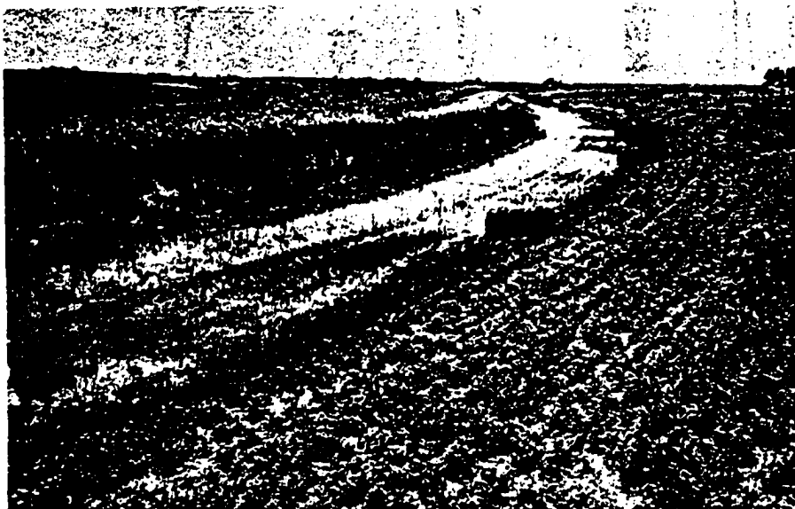
Figure 4. These grassed backslope level terraces near Wiota, Iowa held back water from 12 inches of rain which fell in three days. The water soaked in slowly, reducing runoff and flooding. (Courtesy U.S. Soil Conservation Service)
